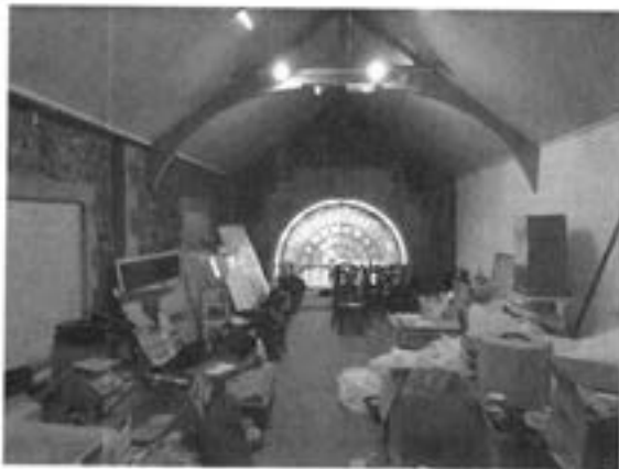
Photo: 1 View of room looking North
