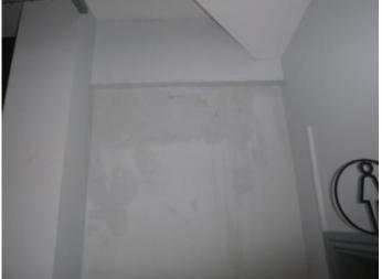
Photo 2.12: Dampness penetrating to the left elevation and migrating through to the entrance foyer
