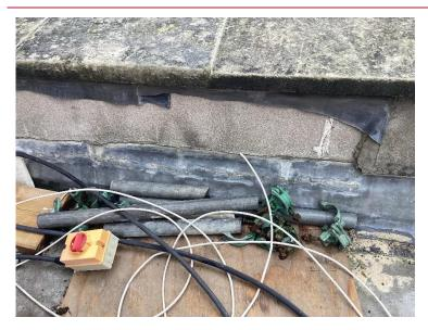
Missing lead flashings at parapet at the  $2^{nd}$  floor roof.
