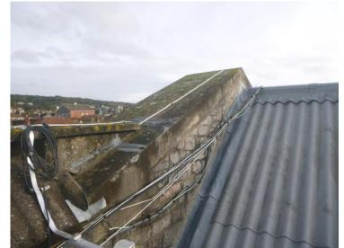
Photo 3.2.6 View of the encapsulated asbestos roof over the Function Room. Temporary Acrypol repairs to cornice junctions.
