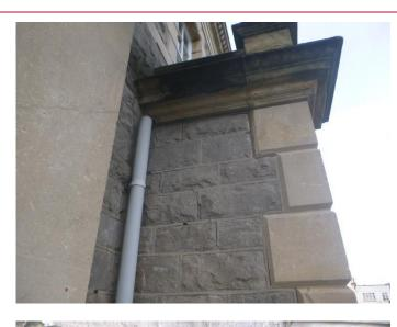
Photo 3.2.2 Rotational movement noted to the bays structure away from the front elevation.
