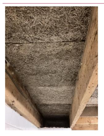
Wood wool slabs form the structure. These do typically provide a degree of fire protection.
