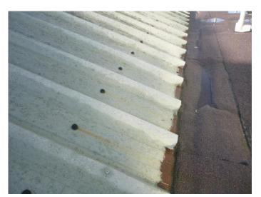
Photo 2.7: View of cut edge corrosion to the metal colour coated roof over the auditorium.
