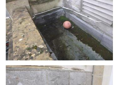
Photo 3.2.4 Spalling surfaces and rotational movement of the bay.
