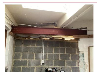
Structural beam. Shuttering for pad stones still in-situ. Allow for boxing in beam or consider fire protection measures.
