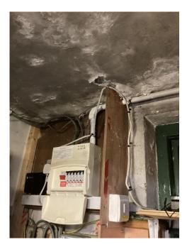
Flaking paint at high level near the door. This could be related to the hopper issue externally.
