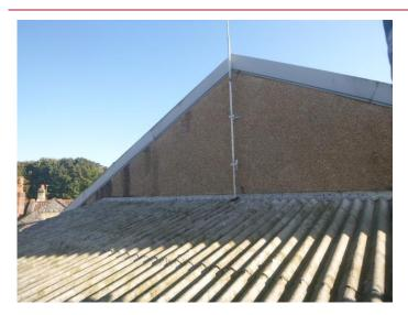
Photo 2.8: View of the rear lean-to roof with asbestos containing material.
