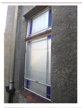
Photo 2.11: Typical metal frame window unit with deterioration evident and unmaintained condition
