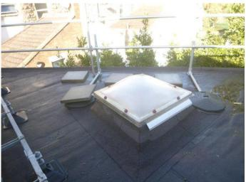
Photo 2.6: Flat roof areas with polycarbonate roof lights prone to ponding rainwater and silting due to poor gradients across the roof.
