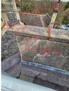
Photo 2.13: Poor detailing at rainwater outlet
