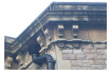
Photo 2.3: Front elevation cornicing with spalled stone eroded and pollution staining. Plastic hopper head and downpipe arrangement has previously been leaking causing stone saturation.
