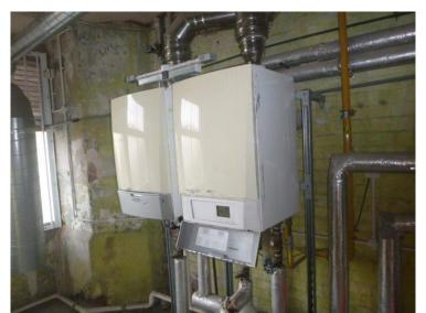
Photo 3.2.7 View of the 2nr gas fired boilers
