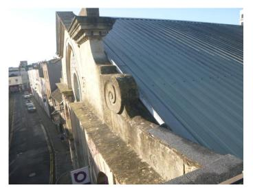
Photo 2.4: View of the front gable pediment and table stone course with general erosion and pollution staining.
