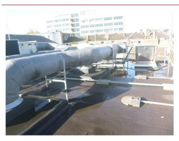
Photo 2.5: Ducted ventilation plant sited on the roof and serving the auditorium and second rehearsal stage room.
