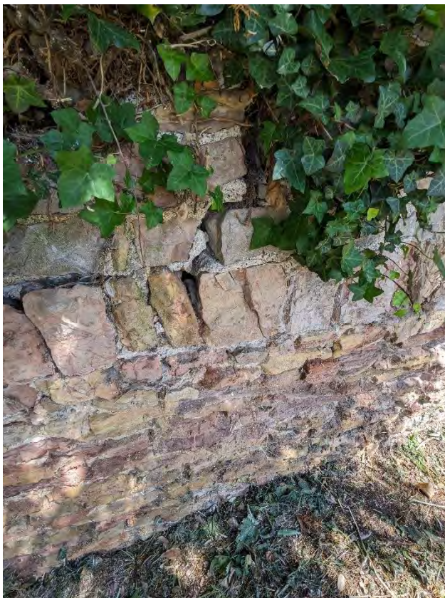
Figure 5: Area of cracking, location shown in Figure 3.
