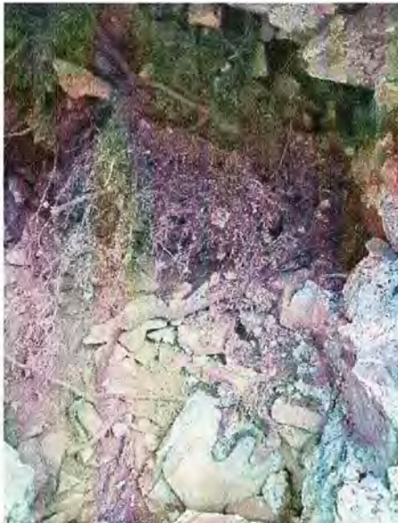
Figure 2: Collapsed wall with root ingress.
