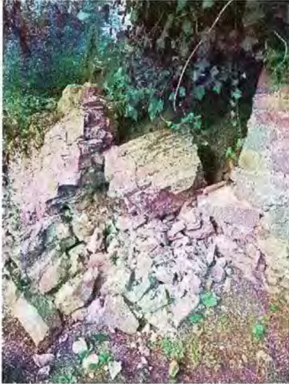
Figure 1: Collapsed wall below T309.
