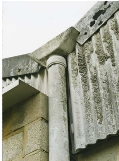
Asbestos cement downpipe, hopper and profile sheet
