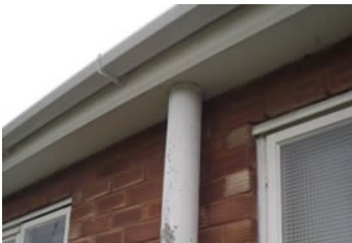
Asbestos cement drainage pipe (downpipe)
